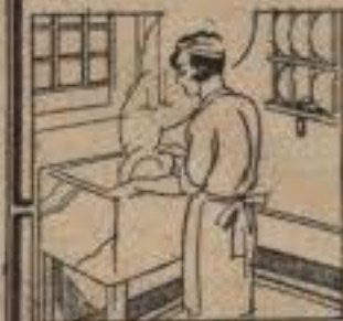
Hot water for washing-up—a constant convenience in the scullery.
